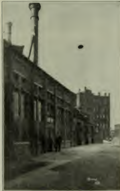
THURGOOD WOOD OF BRIDGE AND BURNES BLDG.
